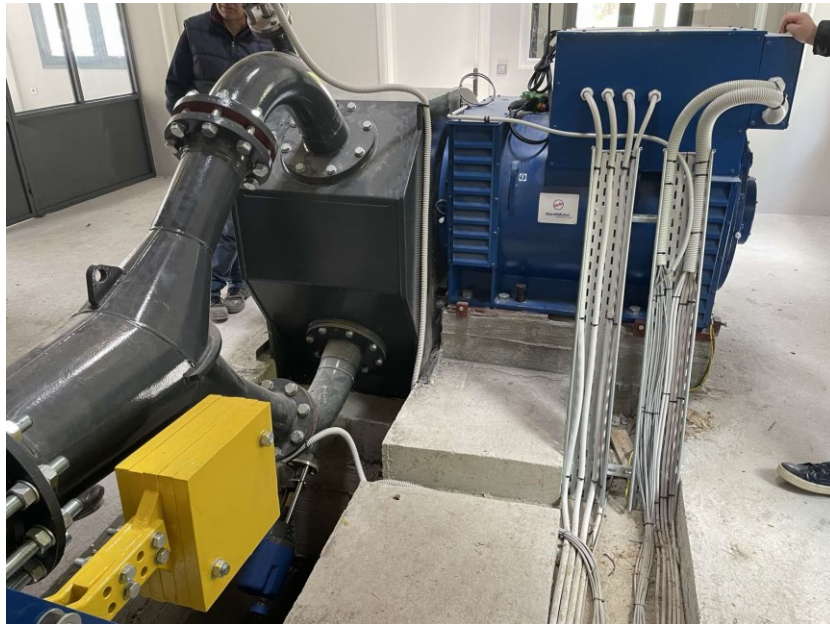
Figure 2.51 Turbin of Hydropower.
