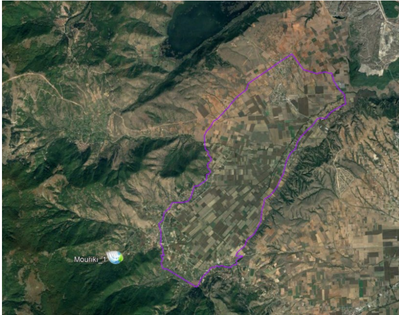
Figure 2.37 Dam of Mouriki basin.
