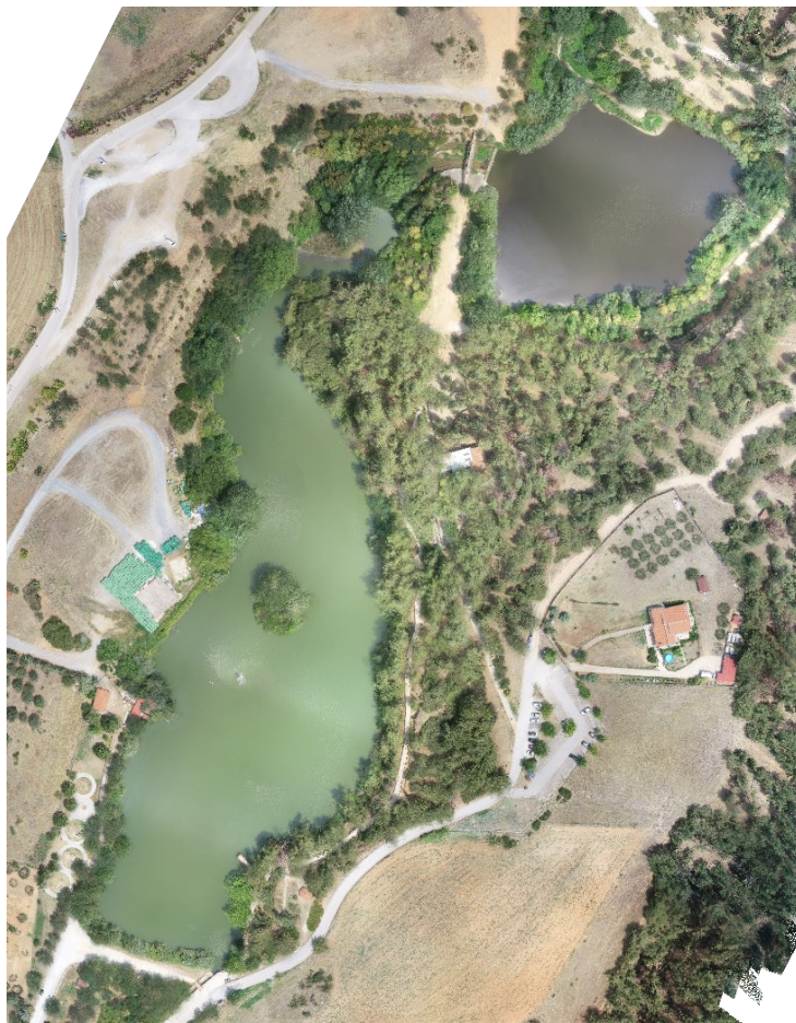
Figure 3.6 Orthomosaic of Thermi dam.
