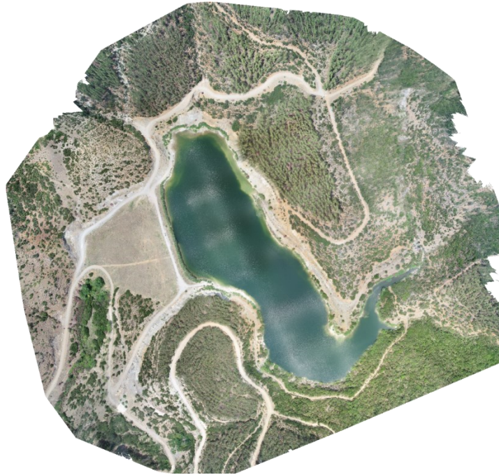
Figure 3.9 Orthomosaic of the Triadi dam.
